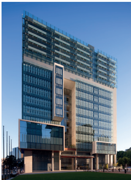
2,500 Lockable dowels were installed on the Supreme & District Court, Brisbane, QLD
