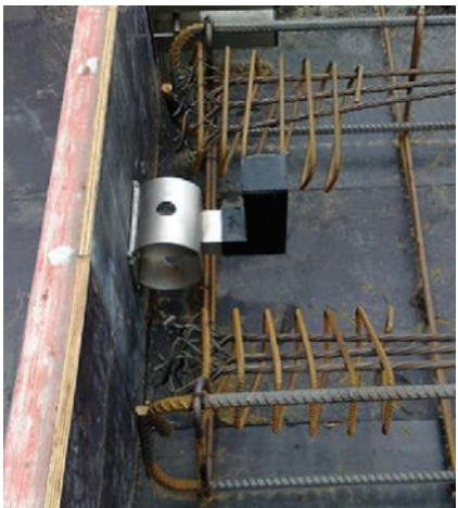
HLDQ-L30 Sleeve nailed to formwork
