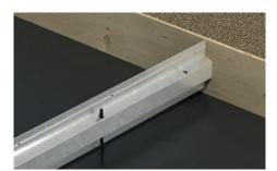
Point key joint in desired location and drive in the supplied pegs. Note that the **longest flange** of the key joint always goes **to the top**.
