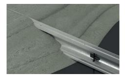
Place the reinforcement and pour the concrete over the key joint. Finish concrete surface to the top of the joint (**not above it**). Always pour concrete evenly to both sides of the joint and ensure concrete is compacted into the keyways.
