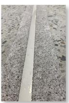
Priming is not normally required. However, demanding applications such as frequently wet conditions or high lift heavy duty applications can be primed with EpiMax 225 for added assurance.
