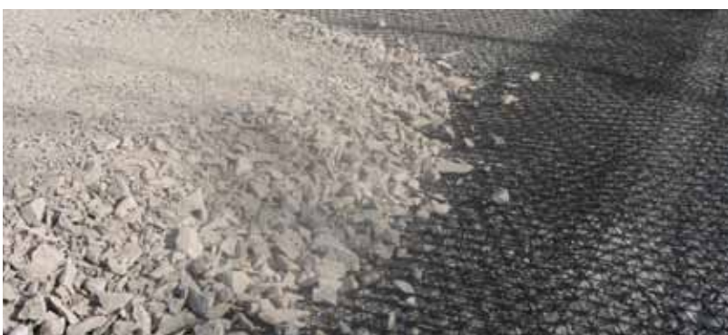
Improving and strengthening the A66 in Melsonby
