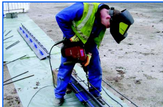
Figure 13. Placing pins.
