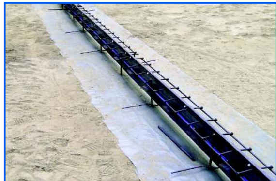
Figure 20. Line of Joints fixed with pins placed both sides.
