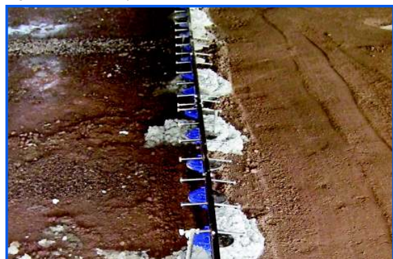
Figure 21. Line of joints fixed with concrete 'dabs'.
