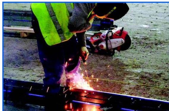
Figure 14. Welding the pins.
