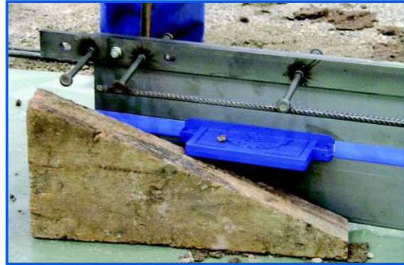
Figure 11. Step 3.2. Adjusting height level
