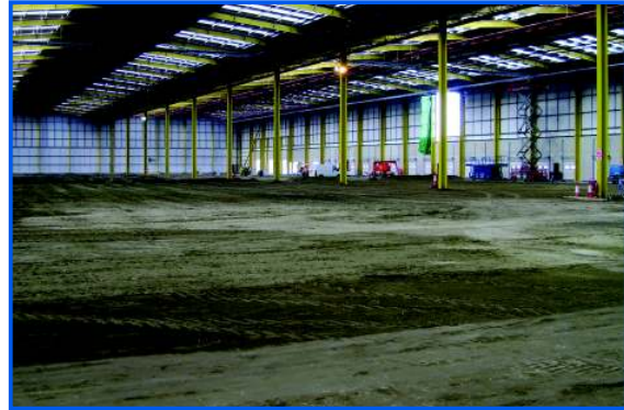
Figure 7. Step 1 - Sub-base level
