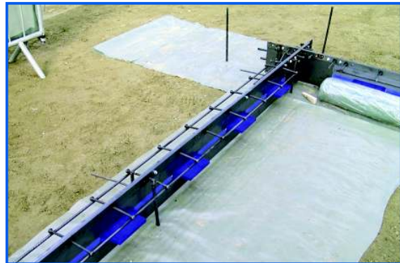
Figure 9. Step 3 - Joint installation.
