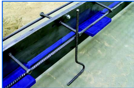
Figure 12. 'T' support as vertical support.
