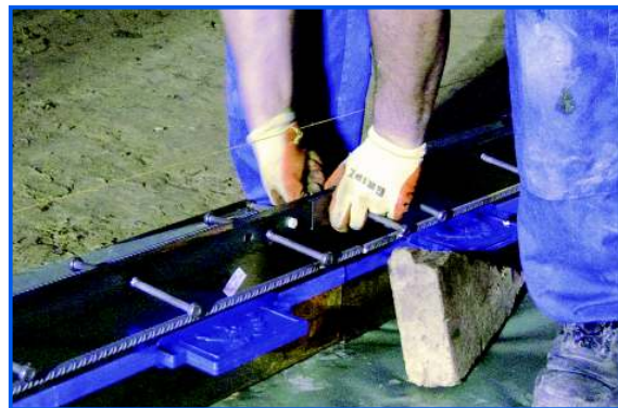
Figure 17. Connecting joints.
