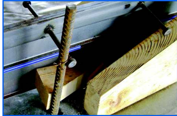
Figure 15. Using timber spacers
