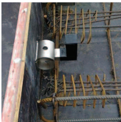
HLDQ-L30 Sleeve nailed to formwork
