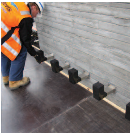
Sleeve pushed over dowel component at core wall
