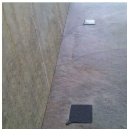
Void formers shown at Slab-to-Wall joint
