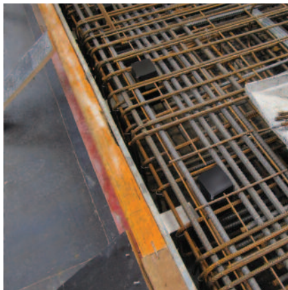
Reinforcement being located around ESDQ-L20 Sleeves
