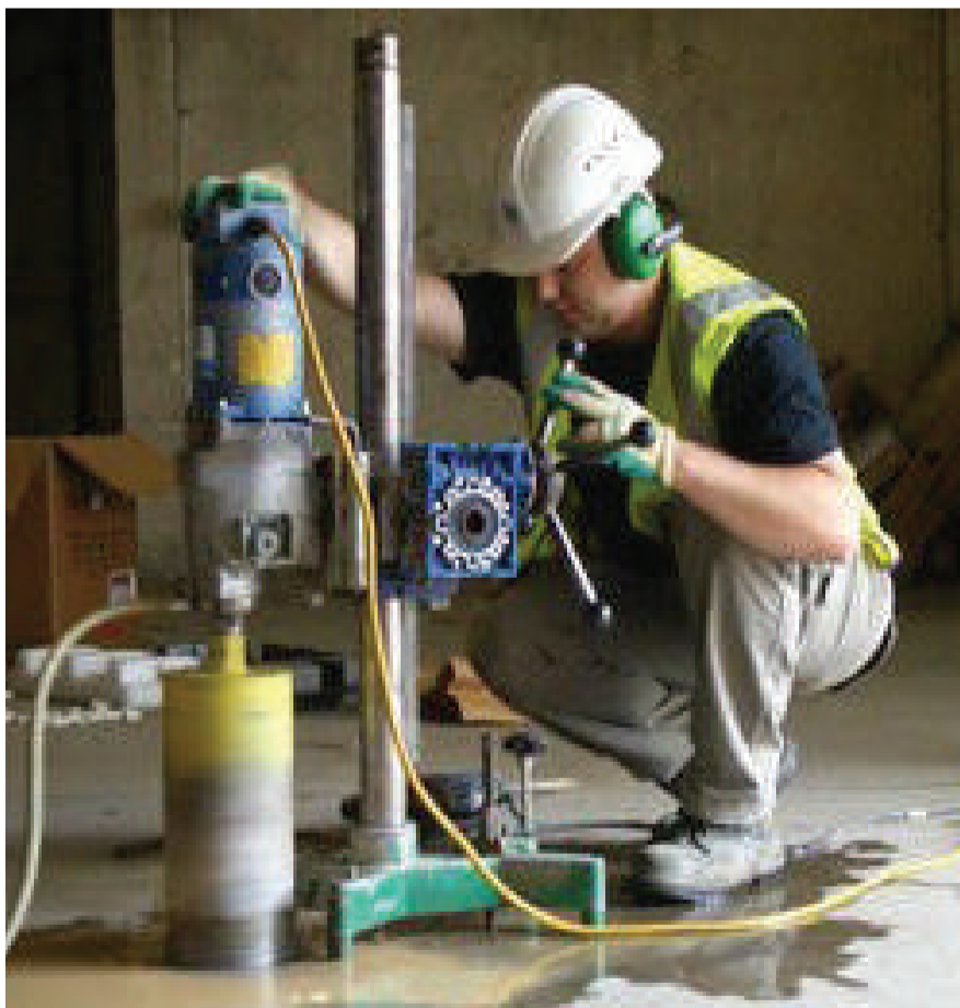
Figure 1-5: Drilled core test [25]
