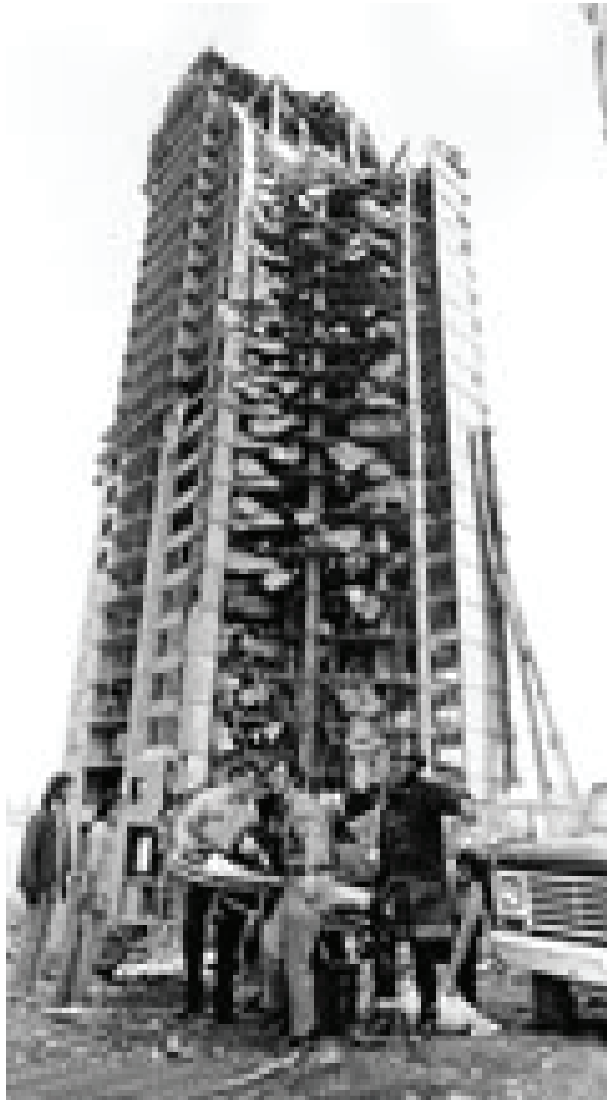
Figure 2-1: Collapse of the Skyline Tower in Fairfax County – 1973 [43]
